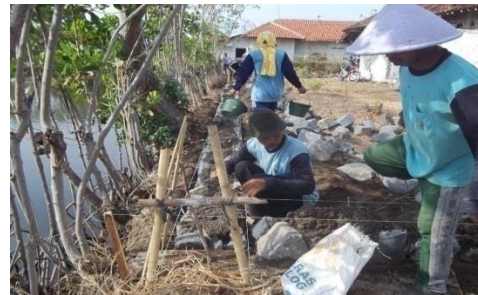
Fig.7 People built the dyke on Kaliwlingi Village, 2014
