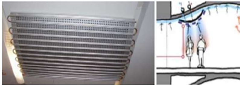
Gambar 2.30 Chilled Ceiling Panel
