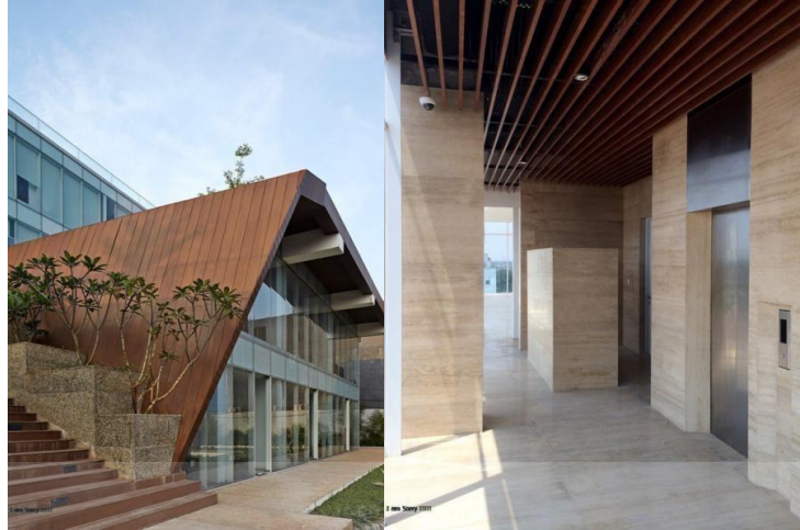
Gambar 2.7 Area Lift Kantor Graha Adhi Media Complex
