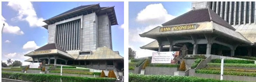
Gambar 2. 7 Fasad & Detail Atap Drop Off Bank Indonesia, Semarang
