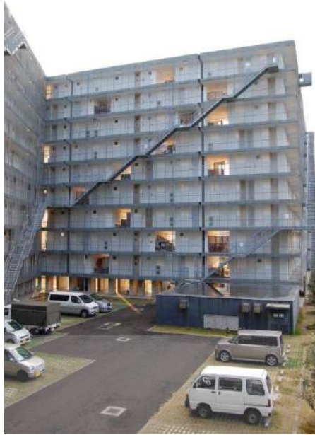
Gambar 2.12 Fasad Gifu Kigata Apartment
