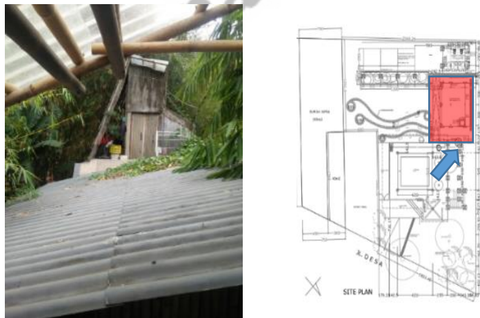
Gambar 3 Material Atap Asbes & Fiberglass Studio Akanoma (Sumber: Data Studio Akanoma & Data Pribadi)
