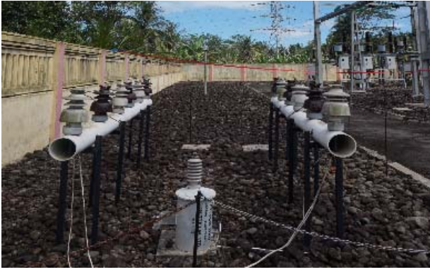
Fig 2. Configuration of insulators aging at coastal area
