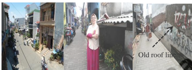
Figure 3.5 Recent housing adjustment (left), low and sinking houses if it cannot be adjustment (middle & right) (Source: survey, 2013)
