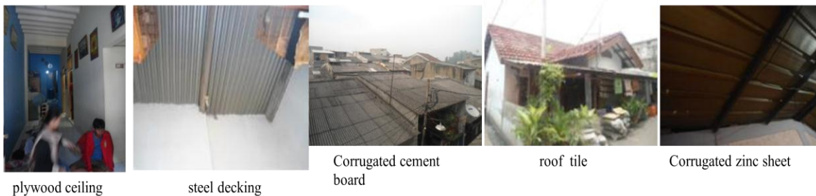
Figure 12. The use of cheap priced light-weight materials for ceiling and roofing
