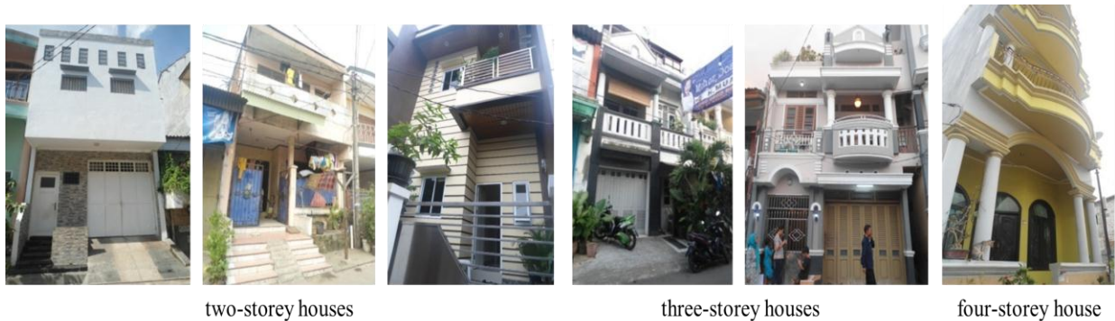
Figure 10. Two or three-storey houses as the results of floor area expansion
