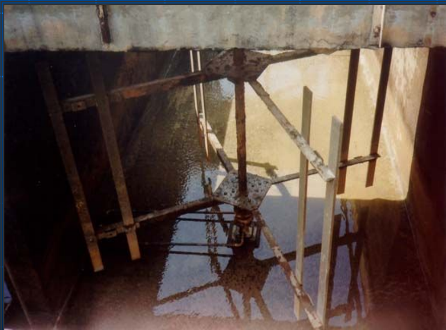
Enlarged View of Paddle Flocculator
