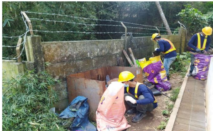
Gambar 3.21 Dokumentasi General Housekeeping
