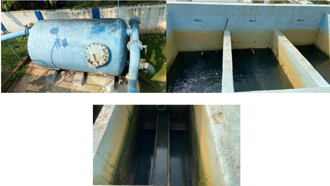
**Gambar 4. 6** Unit Filtrasi IPA Konvensional Perumnas
