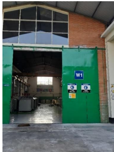
Gambar 5. 1 Bengkel Workshop 1 (W1) “Pekerjaan Eletrikal”
