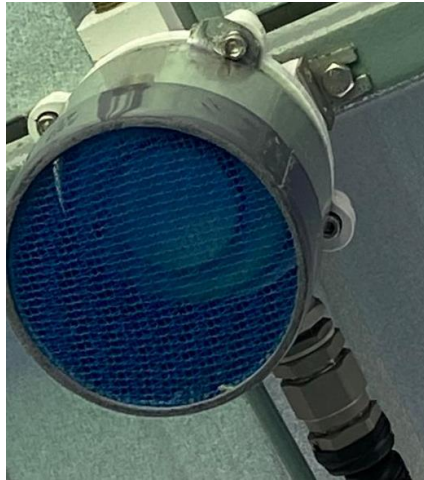
Gambar 5. 8 Smoke Detector in Hazardous Shelter
