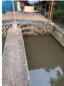
Gambar 4. 6 Coarse Screen
