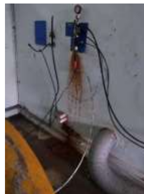
(b) Flow Meter Gas klor
