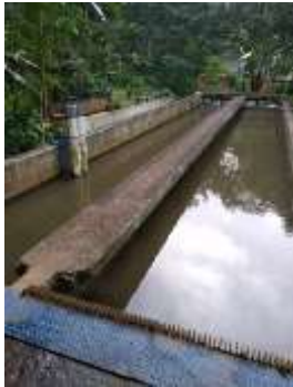
Gambar 4. 5 Unit Prasedimentasi
