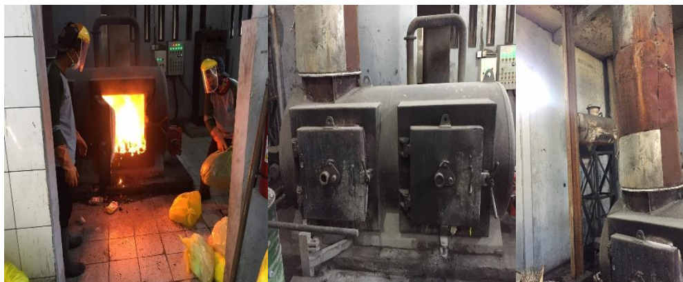
Gambar 4.9 Pengoperasian Insinerator dan Wet Scrubber
