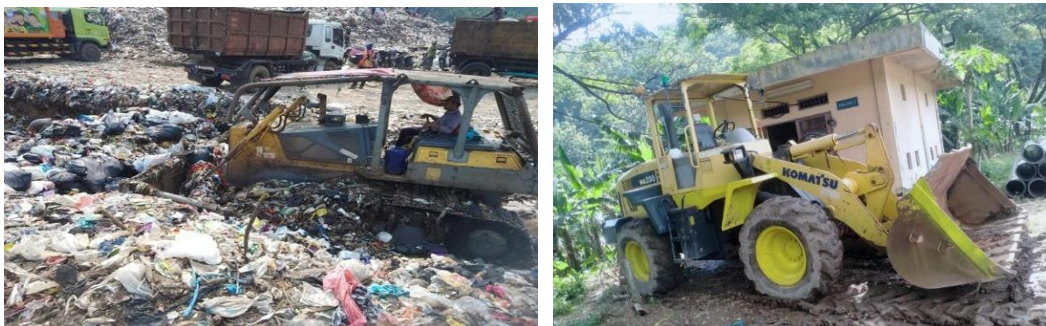
Gambar 4. 8 Bulldozer dan Wheel Loader
