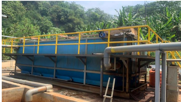
Gambar 4. 17 Dissolved Air Flotation di IPL TPA Sarimukti
