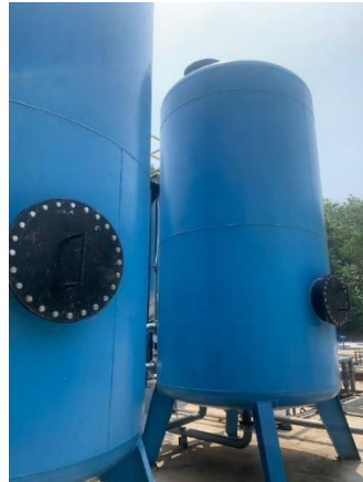
Gambar 4. 20 Sand Filter dan Carbon Filter di IPL TPA Sarimukti
