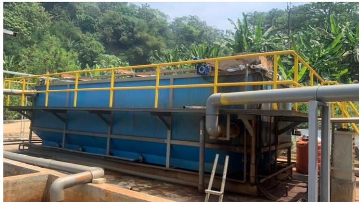
**Gambar 4.9** *Dissolved Air Flotation* di IPL TPA Sarimukti
