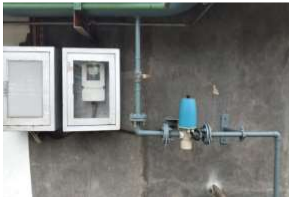
Gambar 5. 21 pH Control Adjustment IPAL PT X
