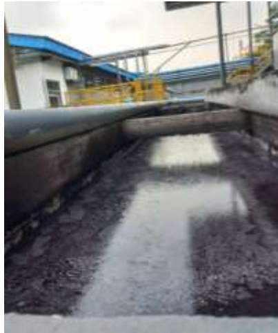
Gambar 5. 19 Transfer Channel IPAL PT X
