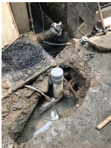
Gambar 5. Pemasangan Access Fitting
