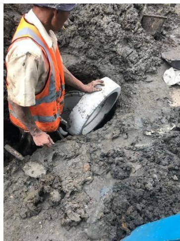
Gambar 6. Proses Pemasangan Manhole
