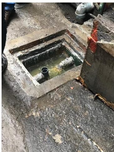
Gambar 7. Pengecekan Grease Trap
