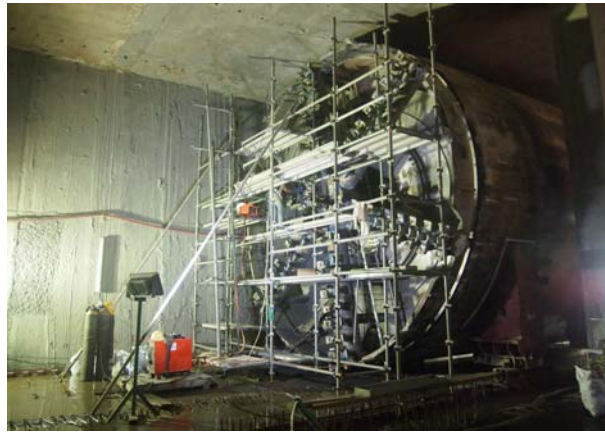
Gambar 1 Mesin bor terowongan ( Tunnel boring machine ) [foto koleksi penulis, 2006]
