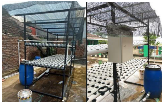
Figure 13. Realization of automation-based hydroponic NFT system
