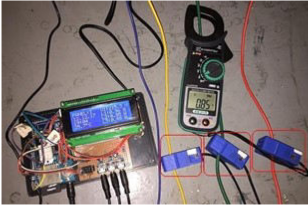
Fig. 15: Three-phase current measurements.
