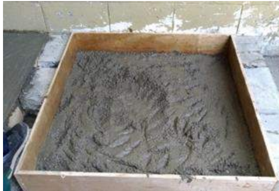
Gambar 6. Proses pengisian lapisan kulit pelat floating concrete
