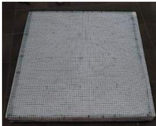
Gambar 7. Proses pengisian lapisan inti styrofoam pelat floating concrete
