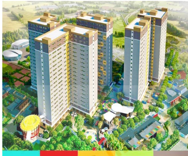
Figure 1. Menara Cibinong Apartment
