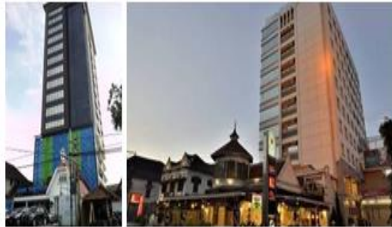
Figure 3. Adaptive re-use of preservation of Historic Buildings in Bandung
