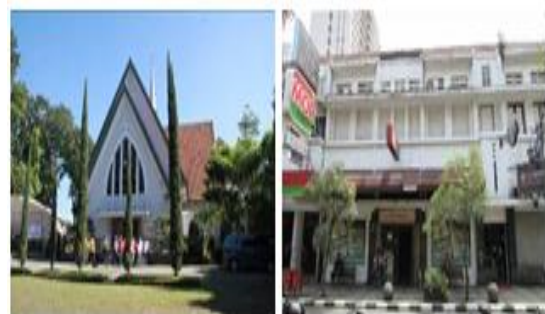
Figure 2. Single and Row Building at Conservation Area in Bandung
