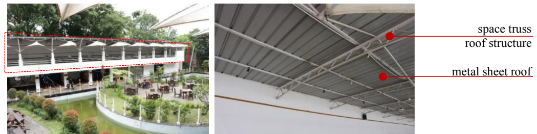
Figure 5. The Roof's Metal Sheets and Membranes of the 2nd Floor of The Centrum's Supporting Buildings at the 2011-2018 Period (Source: Survey and research result, 2017)
