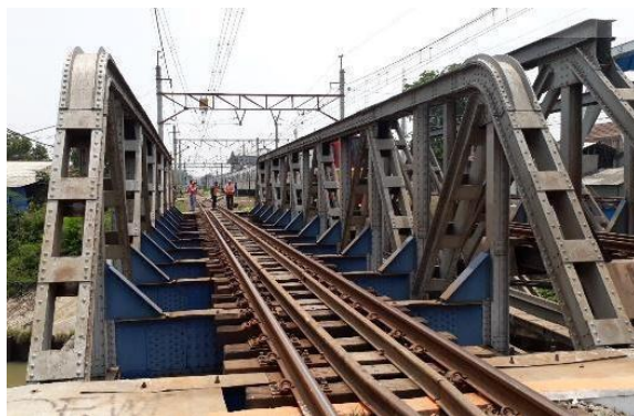
Gambar 2.2 Jembatan kereta api tipe through truss
