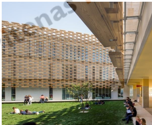
Gambar 2. 5 : View garden The French Internasional School Of Beijing Sumber : Archdaily , diakses pada 18 september 2020
