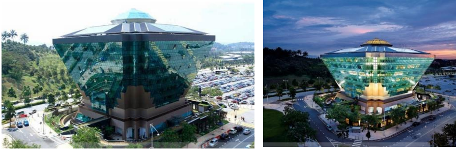
Gambar 2. 3 Diamond Building, Malaysia
