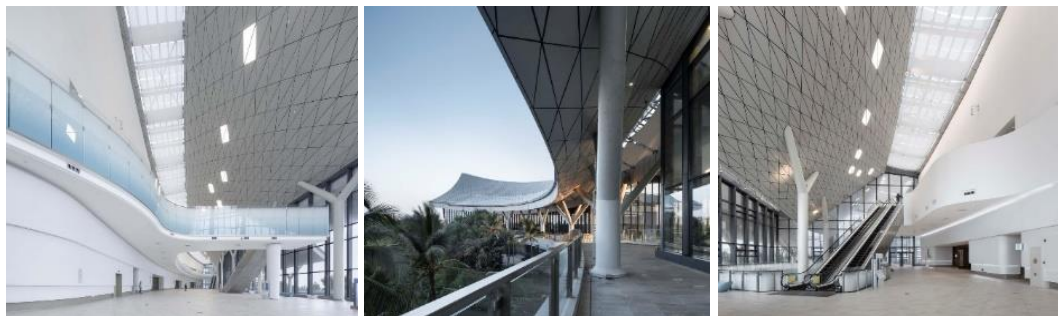
Gambar 2.4 Interior Bangunan China Museum Of The South China Sea
