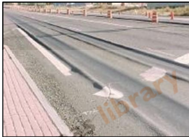
Gambar 2.2 Alur ( Rutting )
