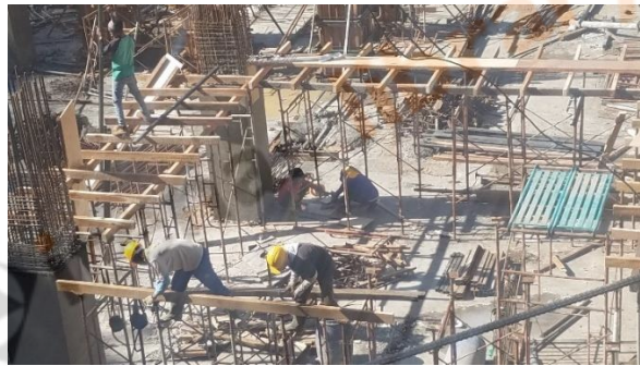
Gambar 2.12 Perancah Tiang Pipa
